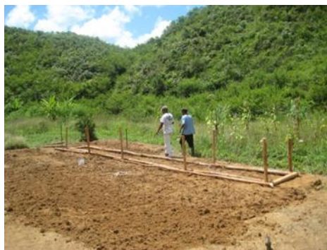
Figure 2. Site preparation of the nursery 40m x 40m
